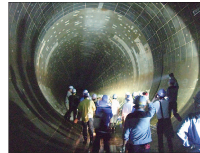
Wada-Yayoi Trunk Sewer (Inspection tour after completion)
