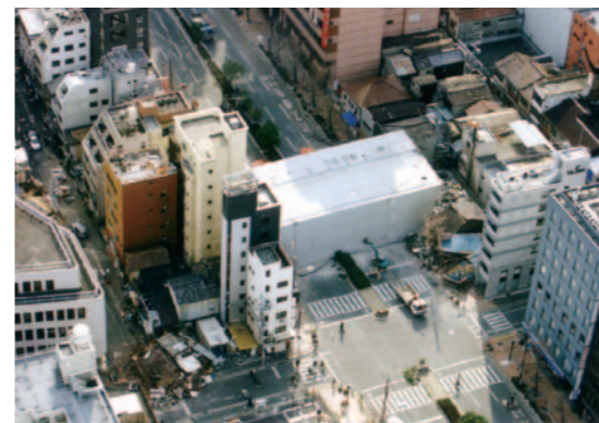
Road blocked by a collapsed building following the 1995 Great Hanshin-Awaji Earthquake
