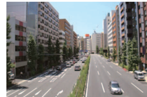
A disaster response route, which will serve as a major artery for the transport of relief, etc. in the event of a disaster
