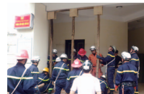
Session for shoring/stabilizing
