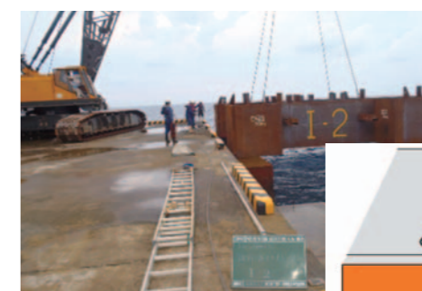
Installation of steel formwork
