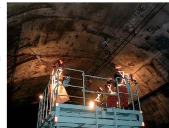
Inspection by sounding concrete
