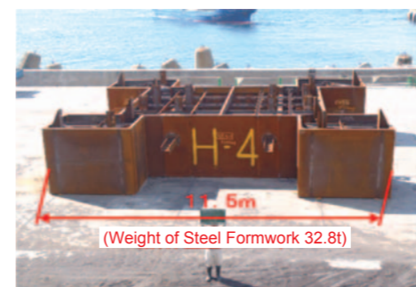
Completed assembly of steel formwork
