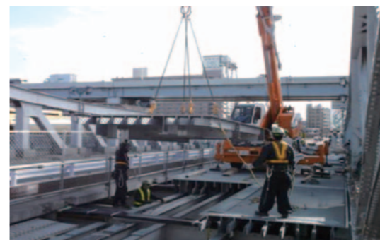
Deck slab replacement (from reinforced concrete to steel)
