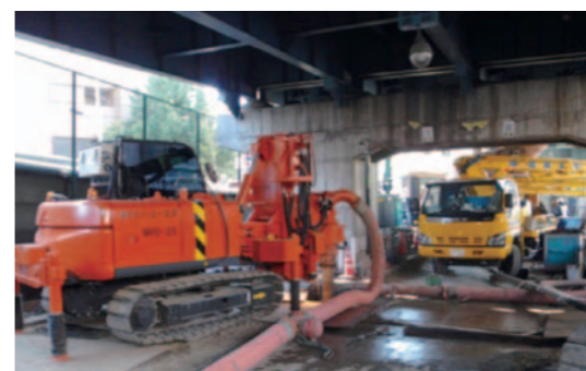
Installation of additional piles
