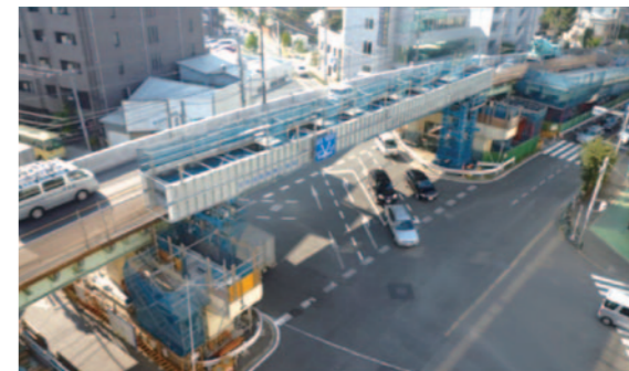
Main girder replacement
