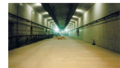
Inside view of immersed units
