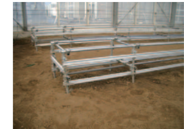
Frame is easily put together using pipes available at retail stores
