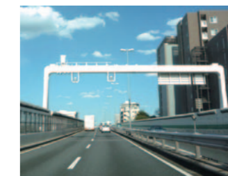
Fixed cameras on an expressway
