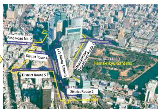
Shiodome area (project underway)
