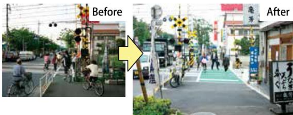
Example of road-widened crossing
