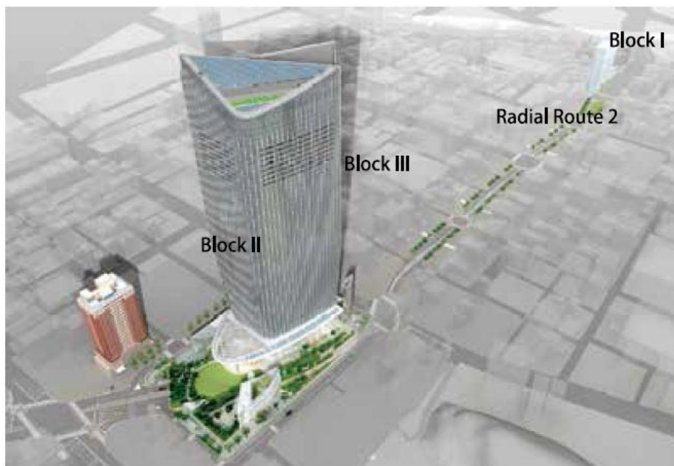
Image of the completed Shimbashi/Toranomon Ring Road No. 2 area
