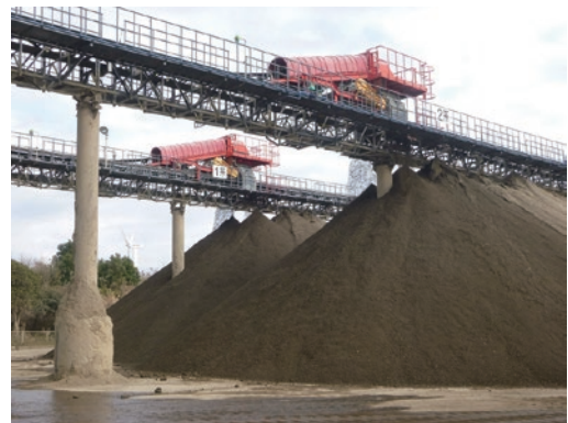
Soil refining plant
