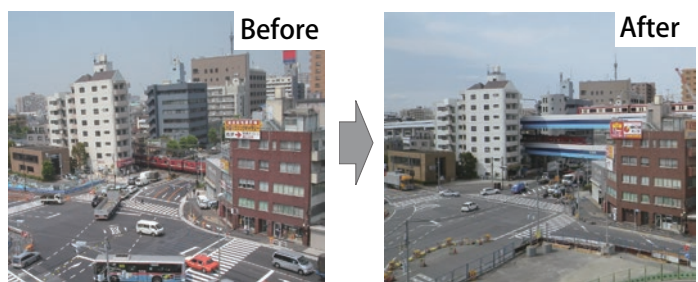
Example of large-scale project for two-level crossings (Keikyū Line near Ring Road No. 8) Photos provided by the Bureau of Construction
