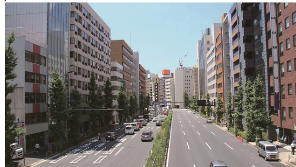
Disaster Response Route to be utilized for the transport of relief, etc., when a disaster strikes
