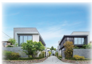
Promotion of enhanced awareness regarding removal of utility poles through urban development
