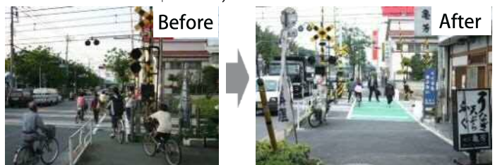
Example of road-widened crossing
