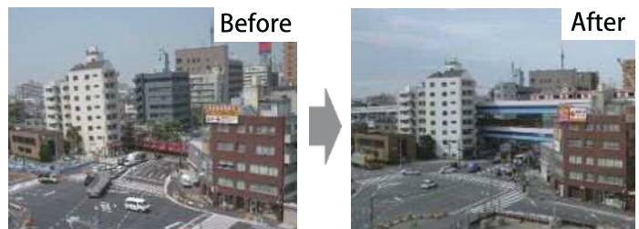
Example of large-scale project for two-level crossings (Keikyu Line near Ring Road No. 8) Photos provided by the Bureau of Construction
