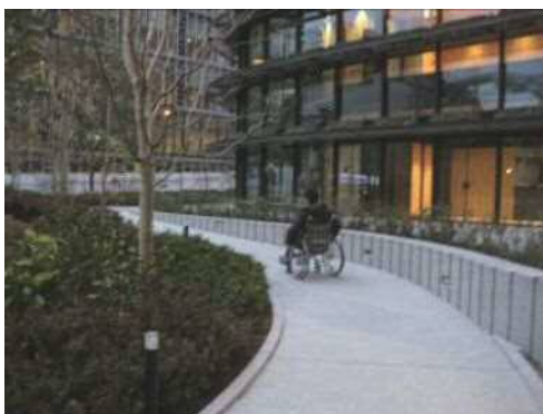
Removing barriers by installing ramps
