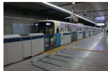
Platform door (Keio Shinjuku Station)
