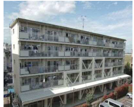
Bracing installed on the balcony side
