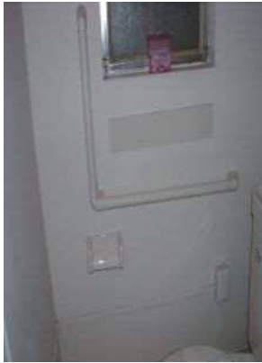
Installation of handrail
