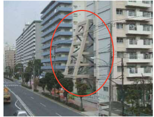
Installation of buttress on the gable wall
