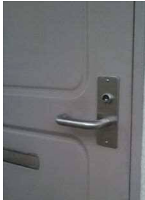
Replacement of door knob with lever handle
