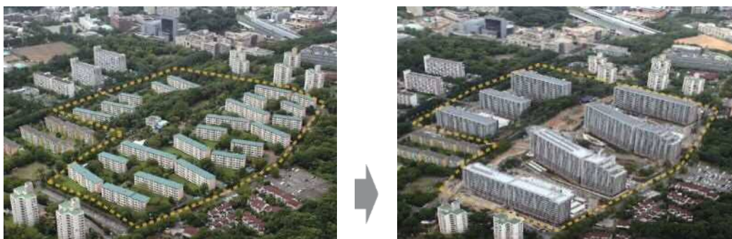
Reconstruction of a large condominium complex
