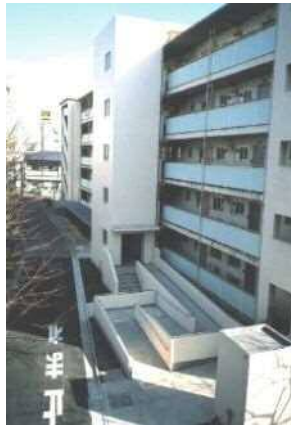
Installation of ramp
