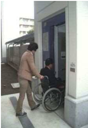
Installation of elevator
