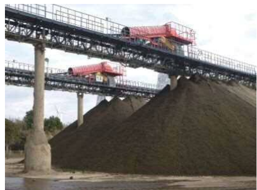
Soil refining plant
