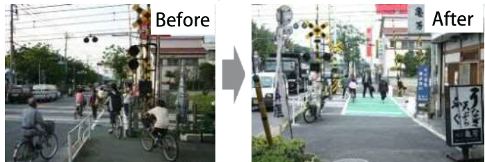
Example of road-widened crossing
