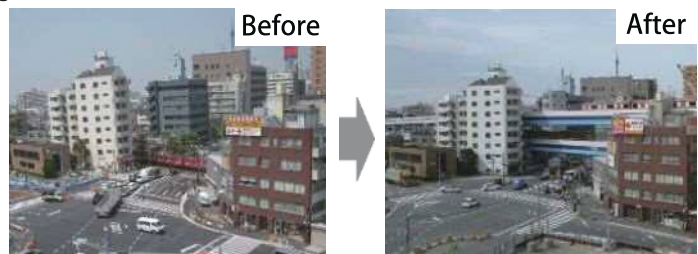
Example of large-scale project for two-level crossings (Keikyū Line near Ring Road No. 8) Photos provided by the Bureau of Construction
