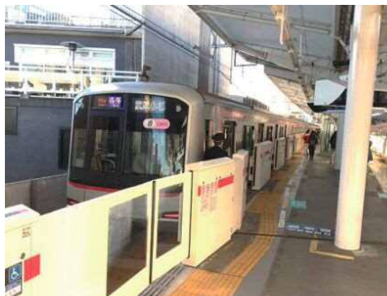
Installation of platform doors (Jiyugaoka Station, Tokyu Toyoko Line)
