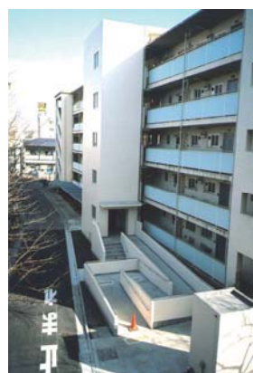
Installation of elevators and ramp
