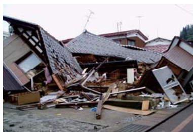
Earthquake damaged wooden houses
