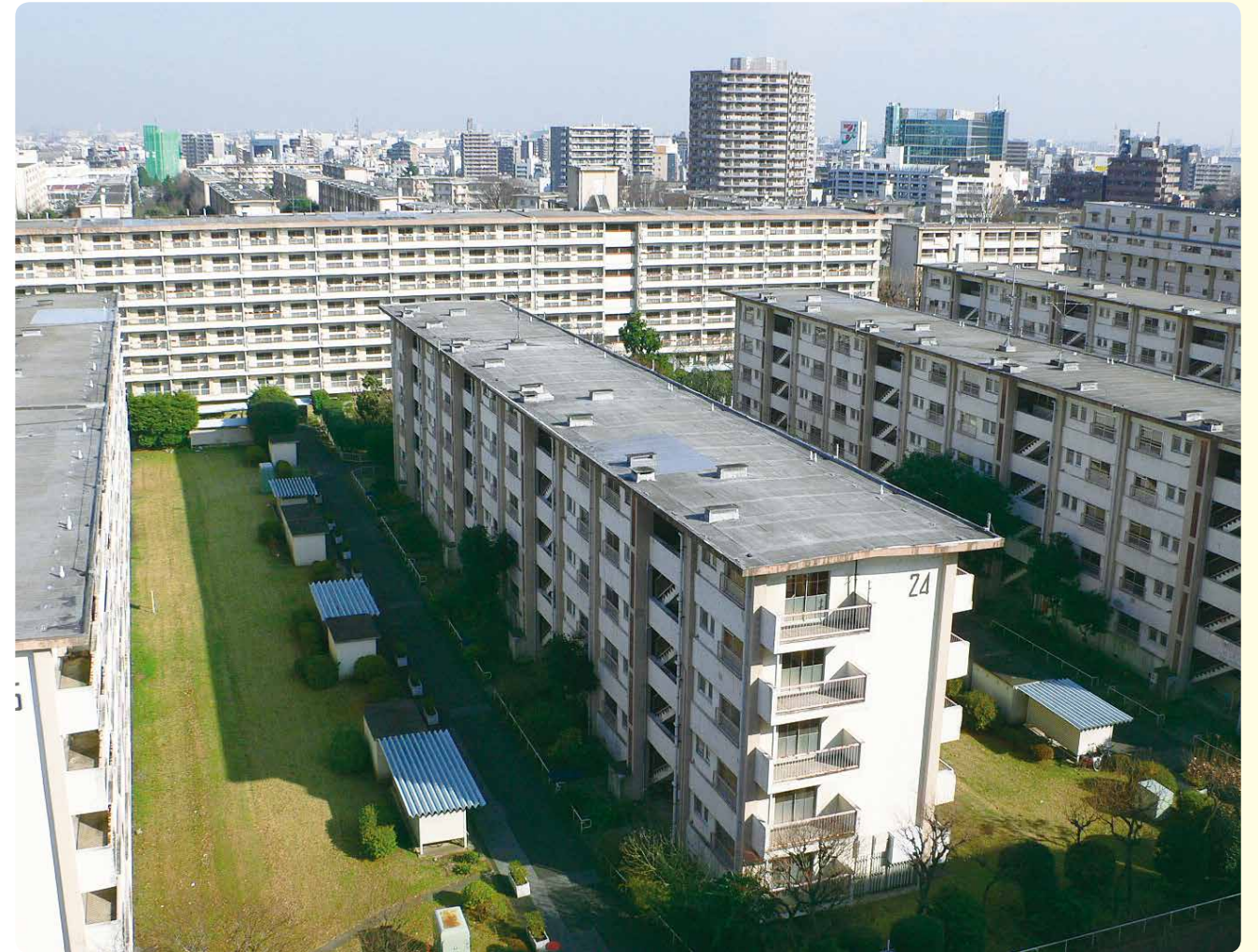
The large Akabane-dai Danchi completed in 1962 shown in a 2006 photo. The development has been rebuilt, and is now named Nouvelle Akabane-dai.
