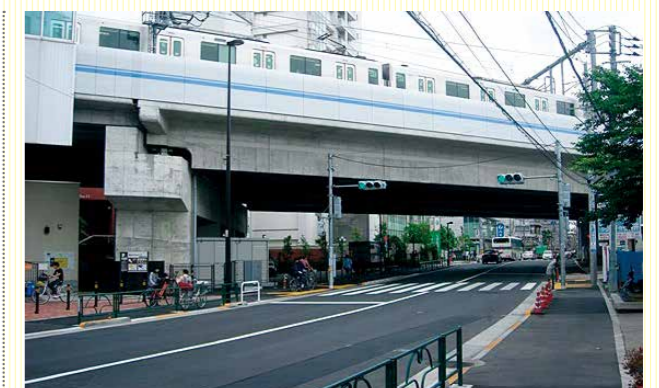
Continuous grade separation project of Seibu Ikebukuro Line Source: Bureau of Construction, Tokyo Metropolitan Government.
