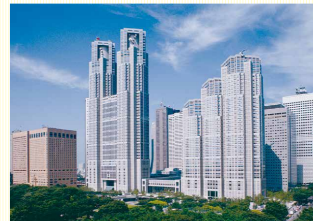
Tokyo Metropolitan Government buildings The current Tokyo Metropolitan Government buildings were designed by Kenzo Tange and completed in 1990. The observation deck on the 45th floor provides a panorama view of Tokyo, the Boso peninsula and Mt. Fuji from the height of 202 meters. Source: Tokyo Metropolitan Government official photo archives.
