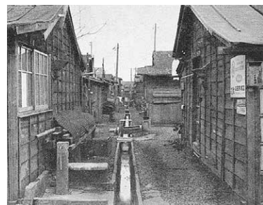
Metropolitan Nishi-Okubo apartment house Shinjuku-ku (late 1940s to early 50s) In the mid-1940s, metropolitan housings were also wooden structures. During the period of high economic growth, large numbers of private wooden rental apartments were constructed and housed the many young people flowing into Tokyo. Source: Jutaku 50 nen shi: jutakukyoku jigyo no ayumi (50 years of housing history: projects of the Bureau of Housing). Bureau of Housing, Tokyo Metropolitan Government.
