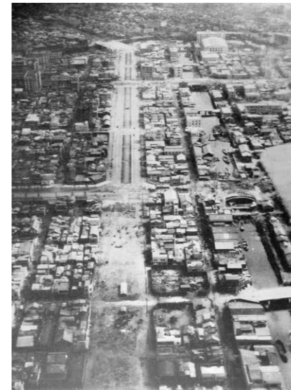
Construction of arterial roads (1930) From Teito Fukko Kinencho (Imperial Capital Reconstruction Commemorative Album), aerial view of Arterial Road No. 1, from the collection of the Edo-Tokyo Museum. Aerial photograph of the area near present day Nihombashi 2-chome, Chuo-ku. Construction progresses on Arterial Road No. 1 (Showa-dori Avenue), road running vertically in the photograph, and Arterial Road No. 3 (Eitai-dori Avenue), road running horizontally near the center of the photograph.
