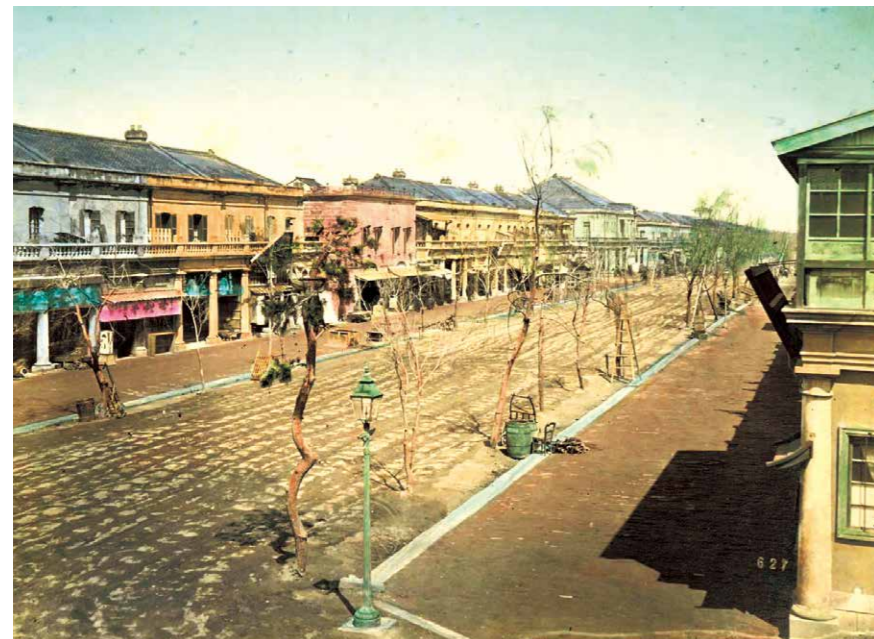
Road with sidewalk (circa 1877) From the collection of the New York Public Library. In Ginza Bricktown, there were three grades of roads, and the height of buildings along the roads was regulated according to the road's grade. With the start of operations of horse-drawn carriages in the built-up area of Tokyo, the separation of roads into streets for vehicles and sidewalks for pedestrians was also planned, and trees were planted between them.
