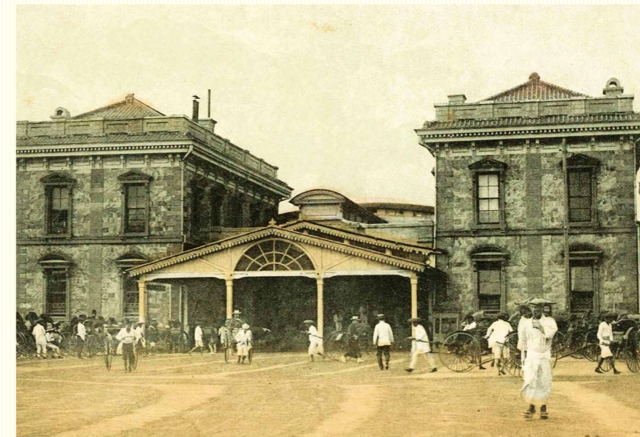
Shimbashi station Tokyo no meisho (Famous Places of Tokyo) From the collection of the Tokyo Metropolitan Central Library. Completed in 1872. Wood and stone western architecture designed by American architect Richard P. Bridgens.
