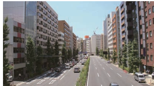
Disaster Response Route to be utilized for the transport of relief, etc., when a disaster strikes
