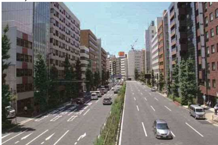
Disaster response route to be utilized in the event of a disaster for the transport of relief, etc.
