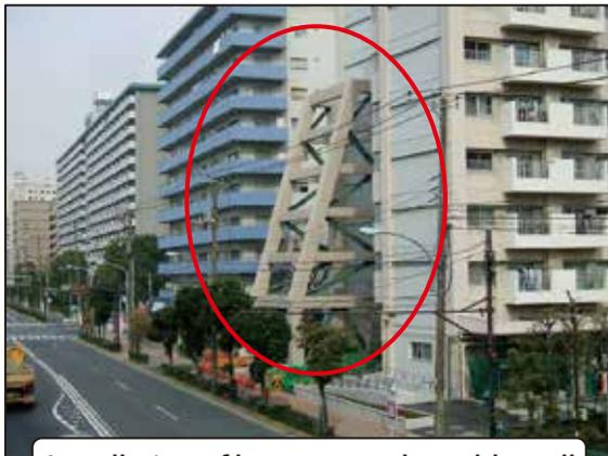
Installation of buttress on the gable wall
